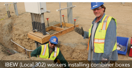
IBEW (Local 302) workers installing combiner boxes
