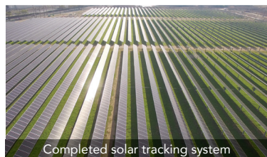
Completed solar tracking system
