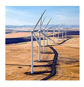
These four wind facilities produce up to 773 megawatts of electricity, enough to meet the electric power demands of approximately 230,000 homes, making PSE the second-largest utility generator of wind power in the U.S.
