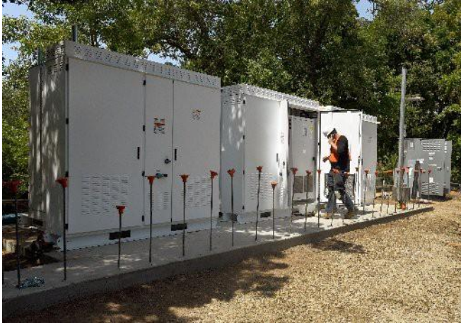
Figure 4: Energy Storage Installation at College of Marin
