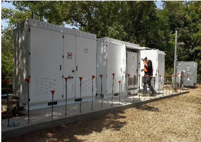
Figure 4: Energy Storage Installation at College of Marin
