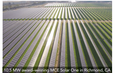
10.5 MW award-winning MCE Solar One in Richmond, CA
