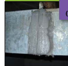
Seal ducts, blow insulation
